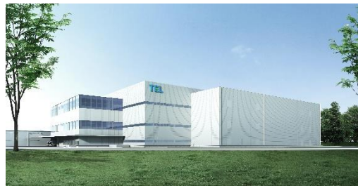
Taiwa-cho, Miyagi Prefecture: approx. ¥47.0B construction cost (Completion scheduled for spring 2025)
